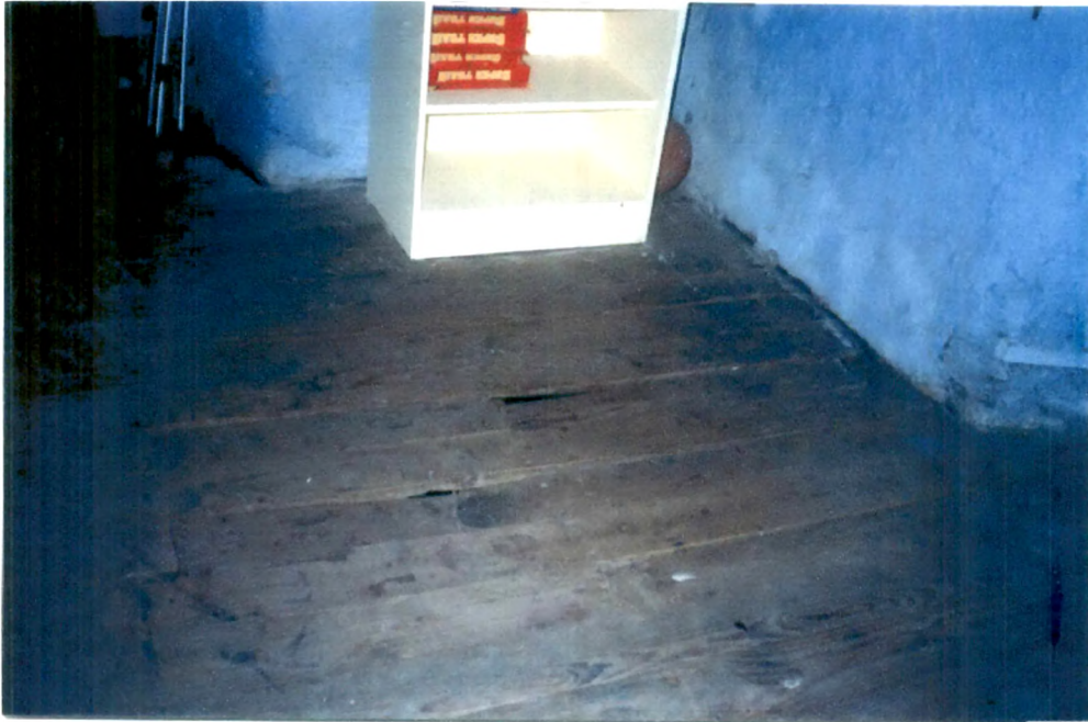
Plate 15: Cracking in Floor made up of Wood
