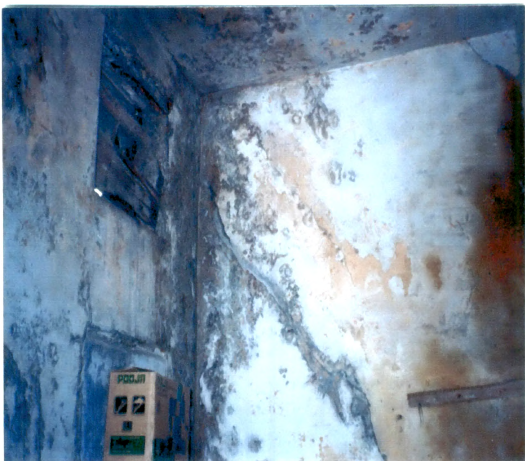
Plate 16: Cracking and flaking off due to dampness in building
