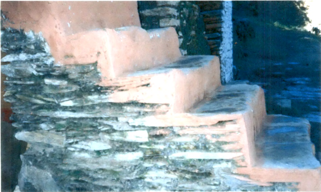
Plate 14: Use of stone in stairs of the house
