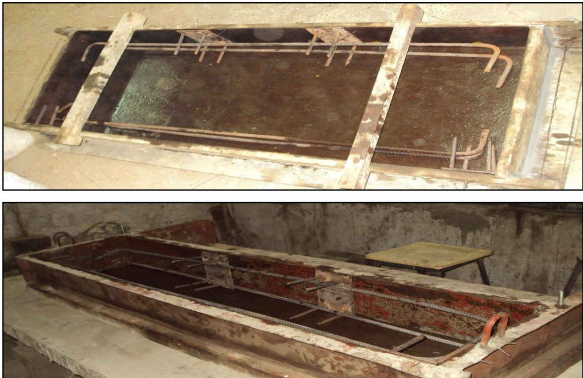
Fig. 3.3 Photographs of Formwork
