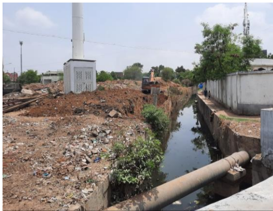
FIGURE 13: CHANNELIZATION IN BHUKHI KAAS NEAR SAMA (D)
