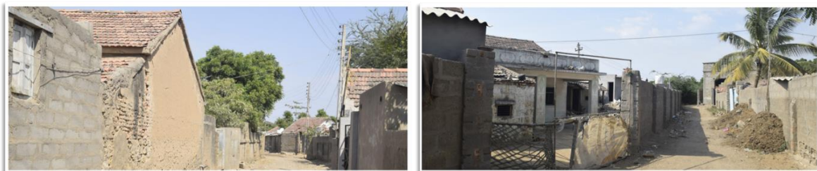
Mud houses replaced by concrete houses
