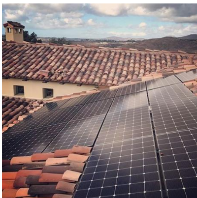
Terracotta roof with solar installation
