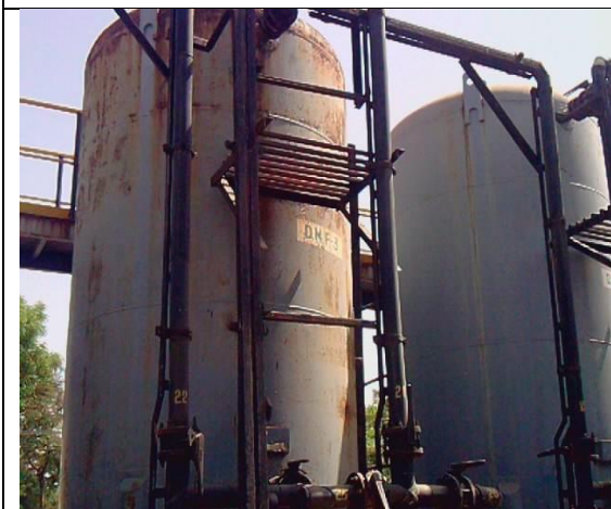
Figure 3.7 Pressure Sand Filter
