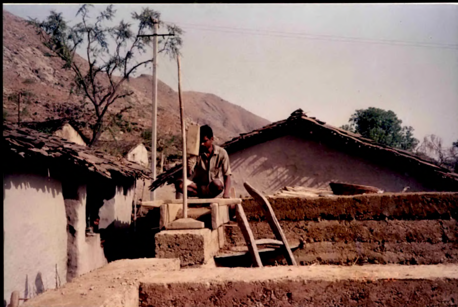
Fg. 8-1 Constructing Clay Walls, Undri, A Bhil, near Udaipur (Study Tour)
