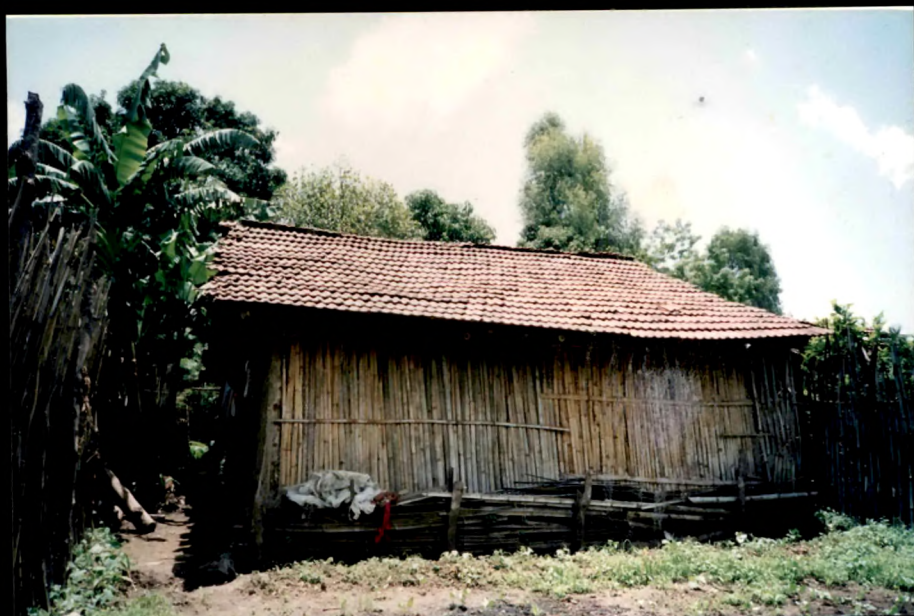
Fg. 21-1 Dhodia Labourer's House Rajendrapur near Waghai, 1993
