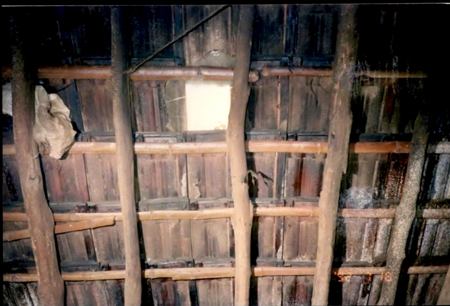
Fg. 18-9 Skylight of a Storage A Konkana House, Malegaon
