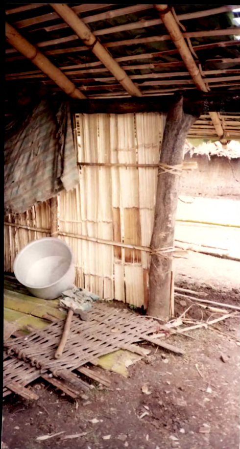
Fg. 19-6 Wall & Bamboo-Mat Floor of a Warli Hut Dongiamba, 1993
