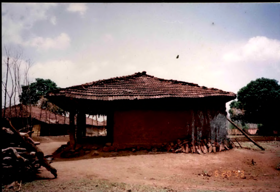
Fg. 18-13 Exterior of Konkana Farmer's House, Pipaldahad, Dangs
