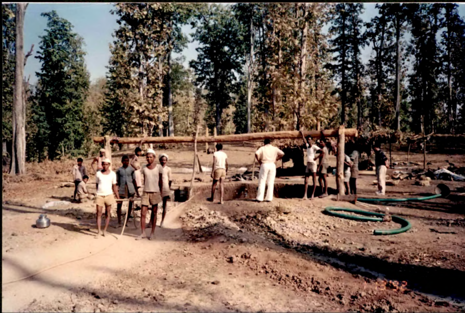
Fg. 52-1 Digging Well, Mulchond
