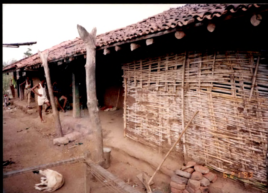
Fg. 20-6 Front View of a Gamit House Kakshala, 1993
