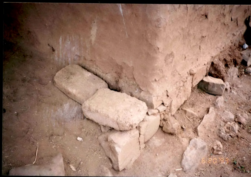
Fg. 18-14 Clay-Block Wall of a Konkana House (details) Pipaldahad, Dangs
