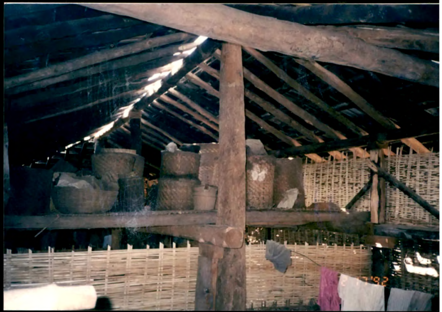
Fg. 18-3 Attic Structure of a Konkana House Borkhet, Dangs, 1993
