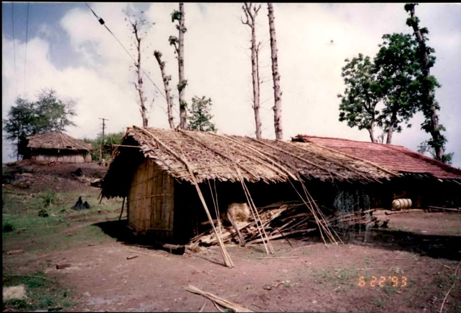
Fg. 22-1 Kotwalia Craftsman's Hut Chichigaontha, Dangs
