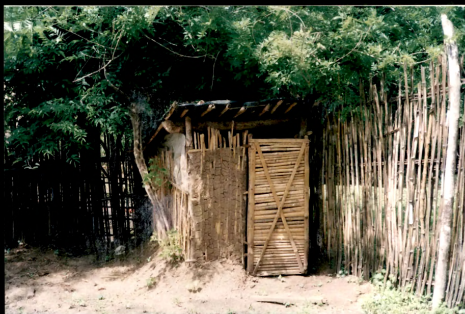
Fg. 21-2 Toilet of a Dhodia House Rajendrapur, Dangs, 1993
