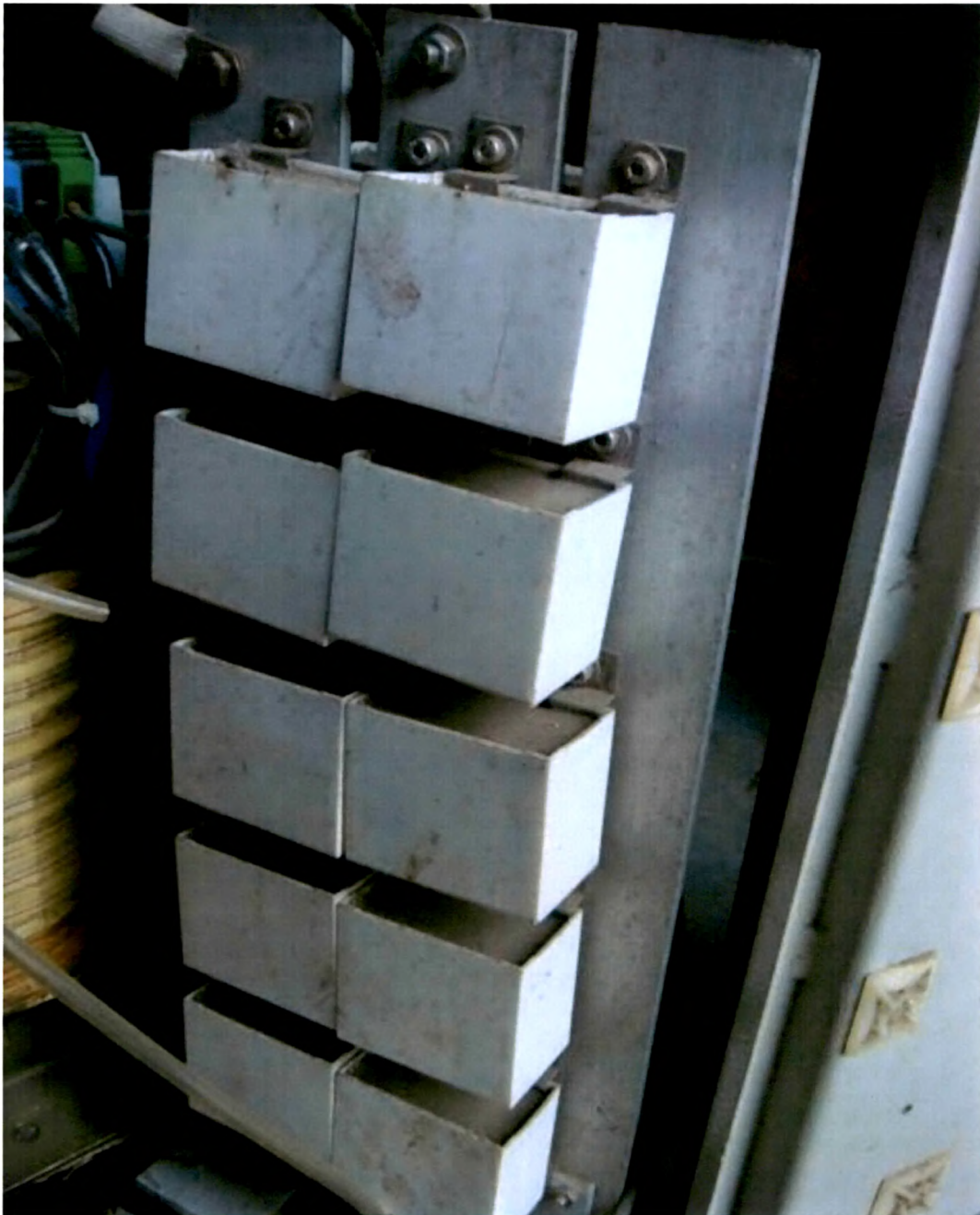
Figure 5-1 Tank Capacitor Bank
