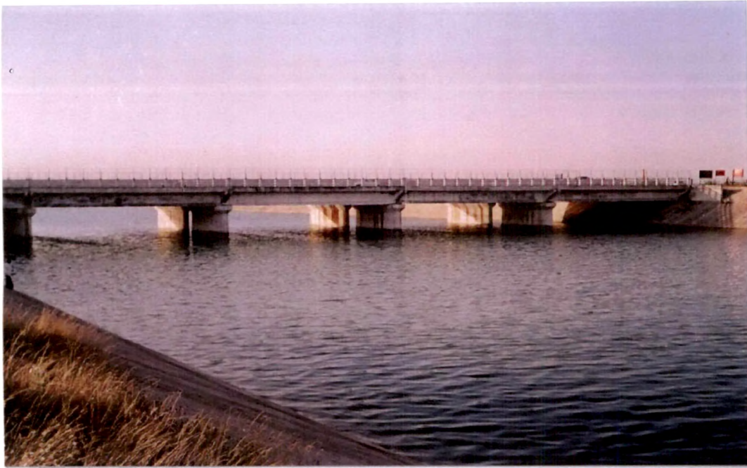
Fig. 4.6 Narmada Main Canal – Source of Surface Water for Irrigation
