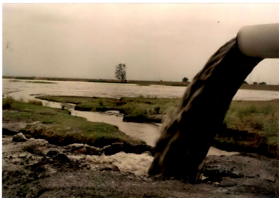
Plate 6.8 Disposal of Coal Ash Slurry From Singrauli STPS In Ash Pond.
