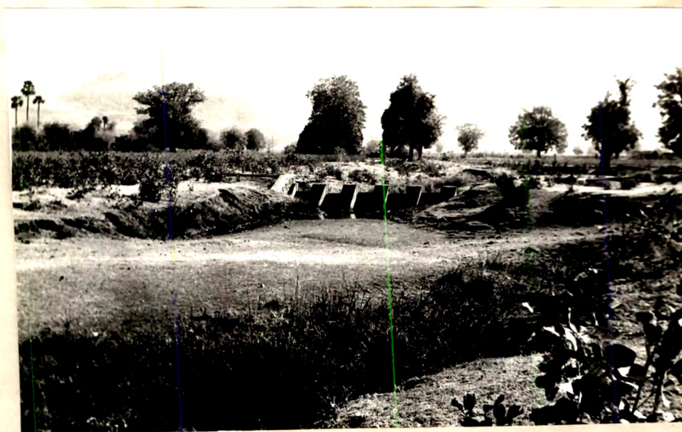
Plate VII.11 Field photograph showing a check dam for augmenting local groundwater potential. (Loc. Near village Untvali).
