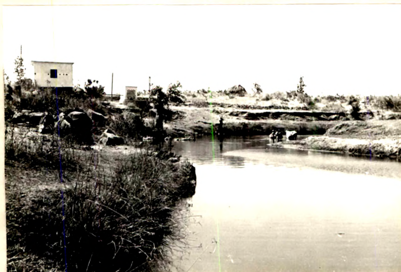
Plate VII.10 Field photograph showing an upstream view of a check dam, enhancing the groundwater yield of the nearby well. (Loc. Near Panvad).
