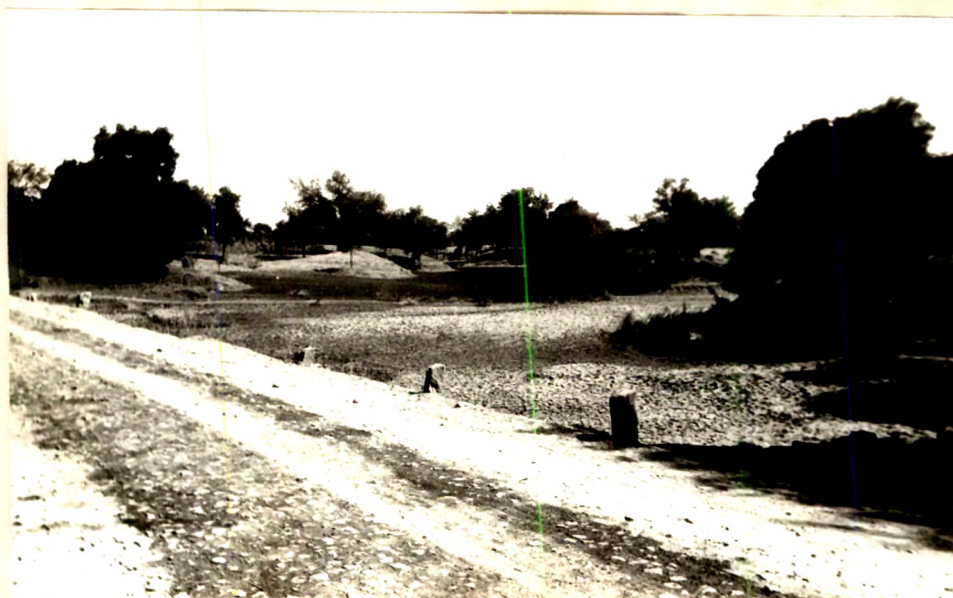
Plate VII.13 Field photograph showing a road embankment creating surface water pool and indirectly enhancing the rate of infiltration for recharging the phreatic aquifer's of metamorphics. (Loc. Near Village Nandpur).
