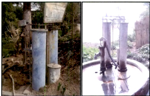
Fig. 4.35: Arsenic Removal Plants (ARPs)
