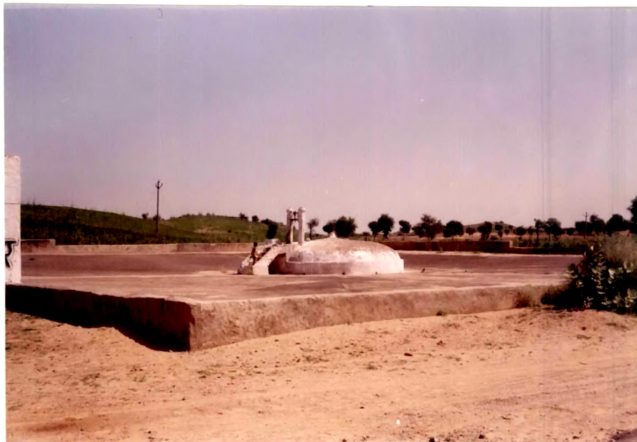
Plate XII.6 Typical tanka (Cistern) made up of concrete structure. Location: Taranagar
