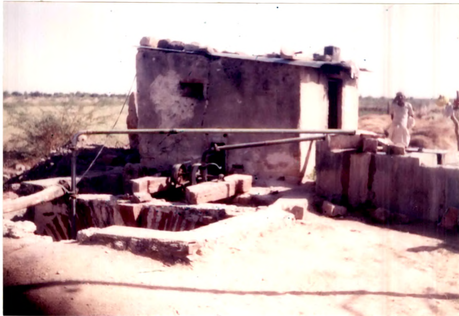
Plate XII.1 A view of lined dug-well in the alluvial plains of Luni river. Location: Alniyawas
