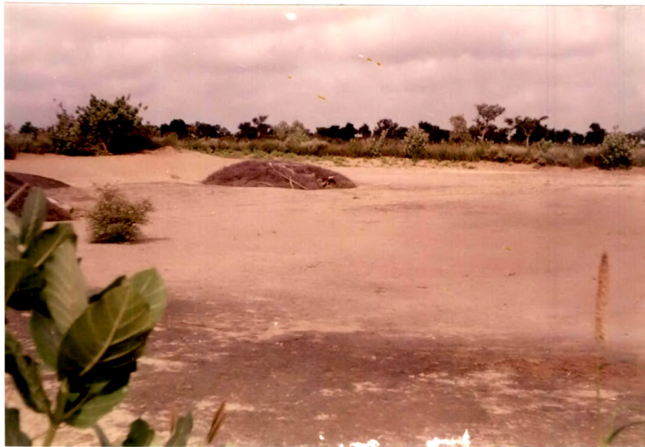
Plate XII.5 Traditional tanka (Cistern) for water storage located in the aeolian terrain around Taranagar-Sardarshaher.
