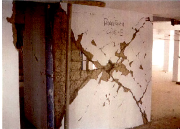
Fig 5.2 Diagonal Shear Cracks in RC Elevator Core
