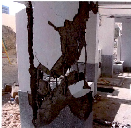
Fig. 5.7 Shear Cracking of Non-Ductile Columns
