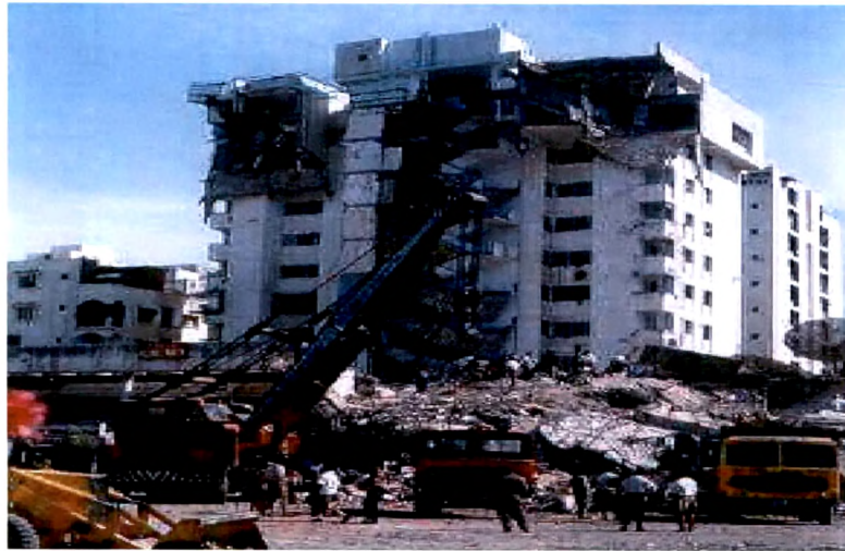
Fig 5.4 Collapse of Flexible Side of Apartment Due to Plan Irregularity
