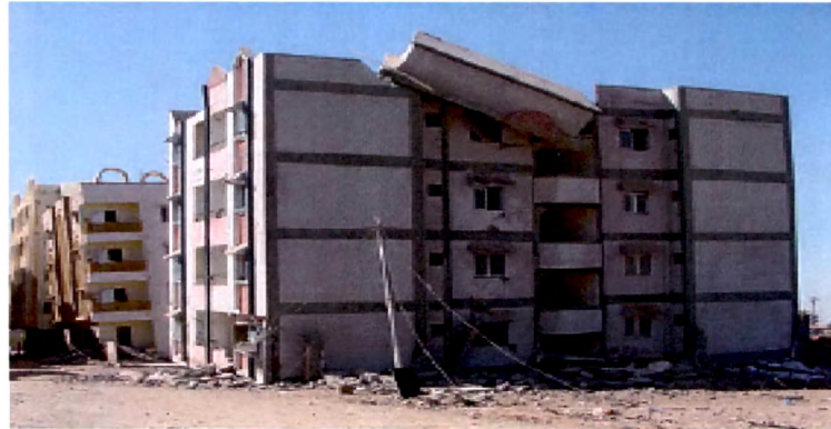
Fig. 5.8 Water Tank Failure
