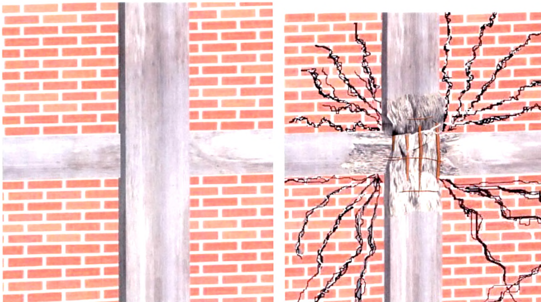
Fig. 5.64 Rendered View of Beam-Column Joint Before and After Earthquake
