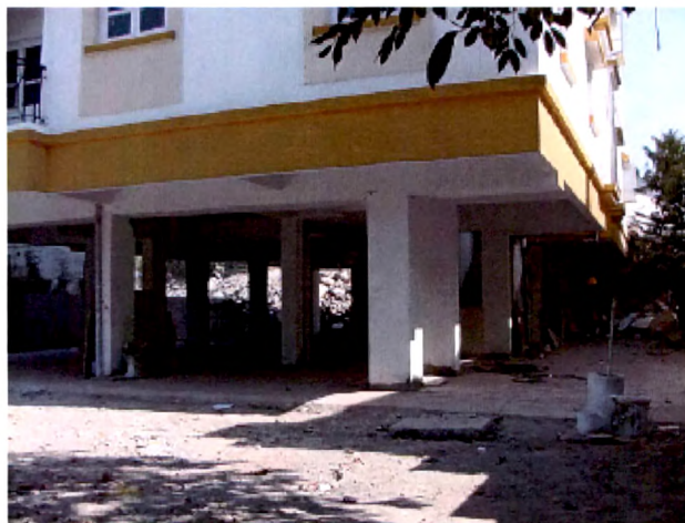
Fig. 5.1 Open Ground Storey
