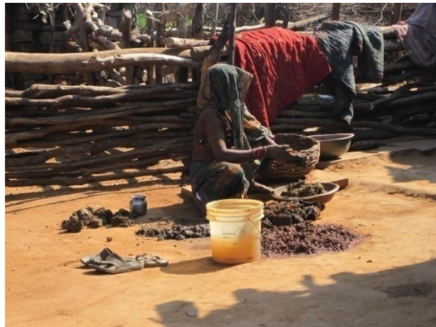
A lady preparing plaster mixture with red sand and cow-dung
