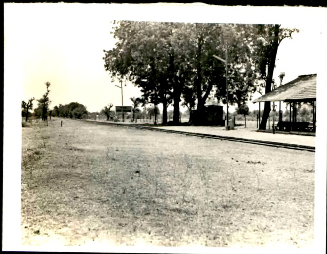
27. Railway station, Bhatpur
