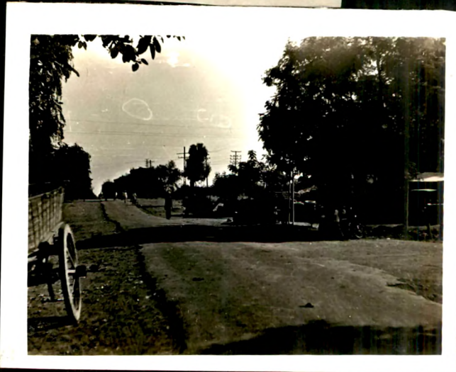
12. Eastern State Highway No. 5 with motor garage & repair shop. Kosindra.
