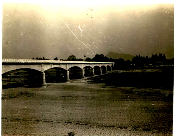
3. Bodali bridge Eastern State Highway No.5
