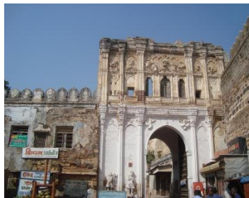
Broken gate to Aaina Mahal
