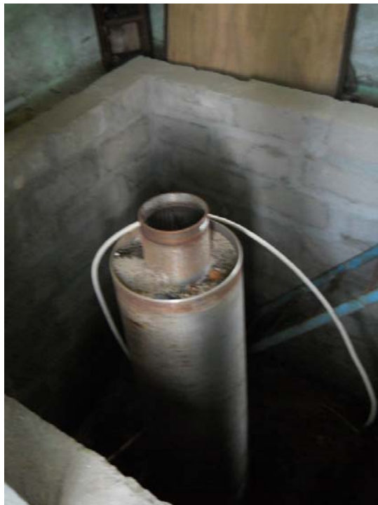
Fig. 6.46 Recharge Bore inside the GWSSB recharge site
