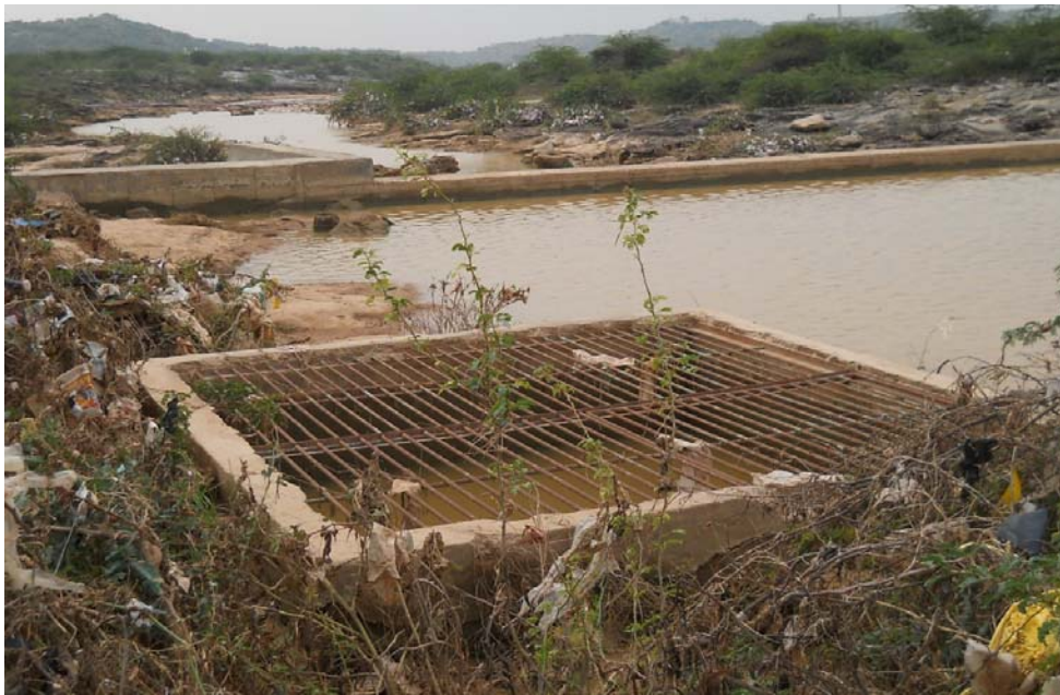
Fig. 6.44 Recharge Tank with Check Dam
