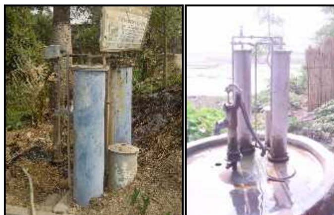
Fig. 4.35: Arsenic Removal Plants (ARPs)
